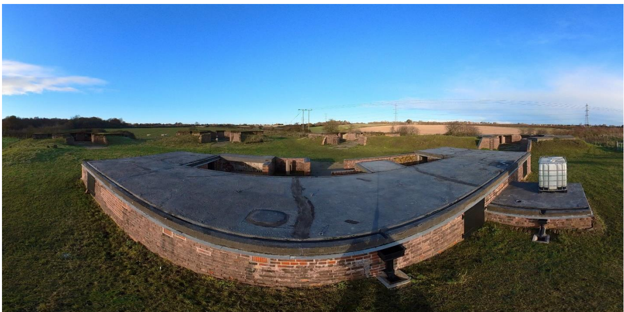
Plate 3 Heavy Anti-aircraft gunsite (1019186) with the command post in the foreground, viewed from southeast (taken with a 360° camera).
